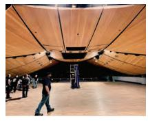
A marvel of engineering, the all-wooden canopy dramatically frames the Jack Singer stage. Weighing over 56 tonnes, it is supported by a series of hydraulic lifts that allow it to raise and lower based on the needs of performers. This canopy is key to maximizing the acoustic potential of the Jack Singer Concert Hall, whether it's for a single soloist or a wall-rattling rock band. To properly assess the condition of the canopy, our contractors modified the side stage speaker attachment points
